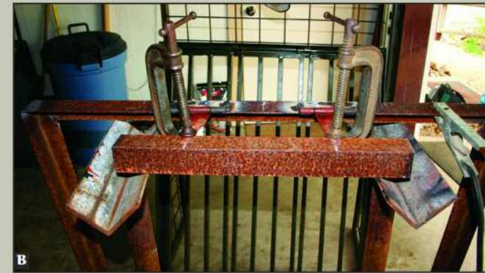
C-clamps secure two T-hinges to the bracket (A). Once secured, a welding machine is used to tack hinges into place. A small piece of angle iron is attached to the other side of the hinges to construct the trigger mechanism (B).
